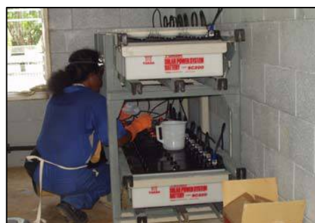
Tino DeBrum wired new parties for the solar system in Namu
